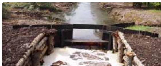
Figure 3-5: More sophisticated (but still low cost) structures on collection drains can be constructed with earth fill and wooden boards (example from United Plantations, Malaysia).
