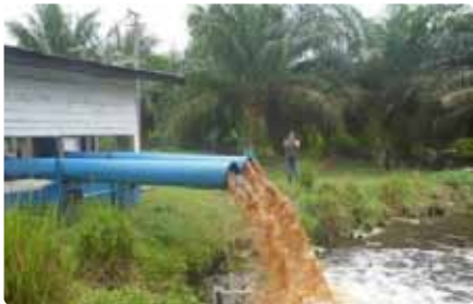
Figure 3-10: Pumping water to a canal to raise water level in particular during dry season.
