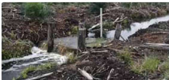
Figure 3-4: Water control structures do not need to be expensive structures and can be simply constructed with wood or sand bags.
