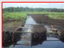
Overflow gate strategically located to discharge excess water into canal system.
