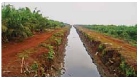
Figure 3-8: Over-drainage in main drain in a peat dome area during dry seasons may result in high CO 2 emissions, subsidence rates, increased risk of accidental fires, as well as significantly reduced yields.
