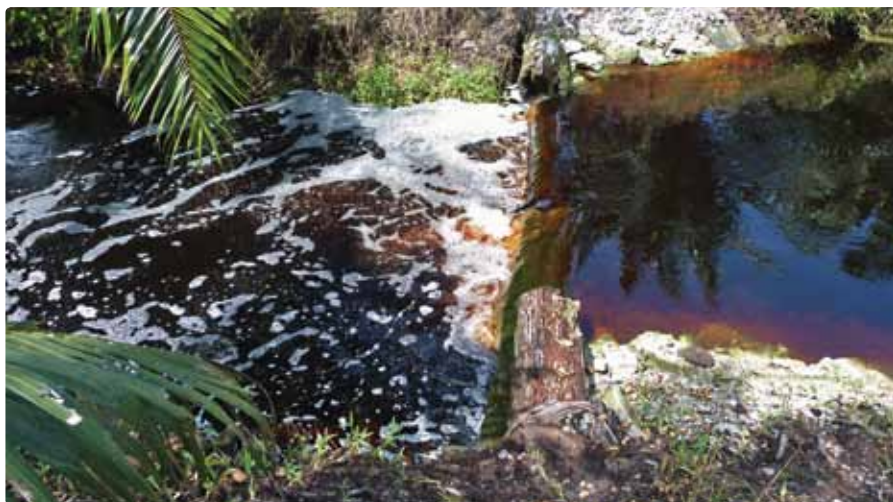
Figure 7-4: One weir installed at every 20 cm drop in water level to enable water retention along collection drains.
