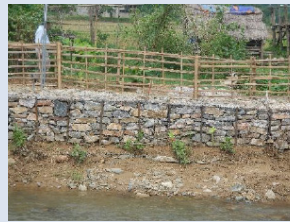
Vegetated gabions wall, one month after construction.
