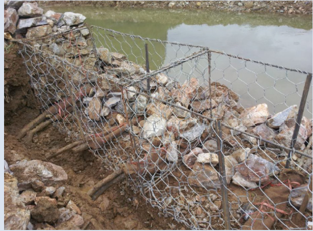
Constructing vegetated gabions.
