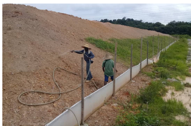
Figure 14: Hydroseeding Technique
