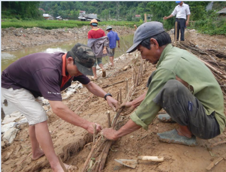
Installing live fences on a riverbank.
