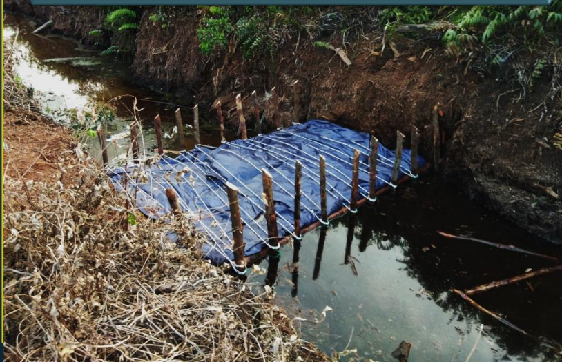
Canal Blocking Construction
