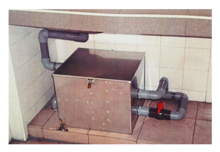
GREASE traps (*pic*) are designed to separate and capture waste fats, oils, grease (FOG) and food waste before they enter the drain and sewers.
