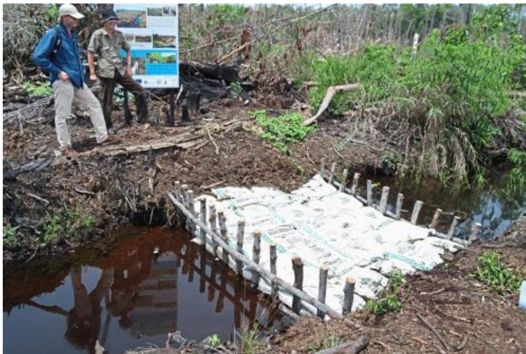
Canal blocking to restore peat swamp's high water table is part of efforts to preserve the unique forests.
